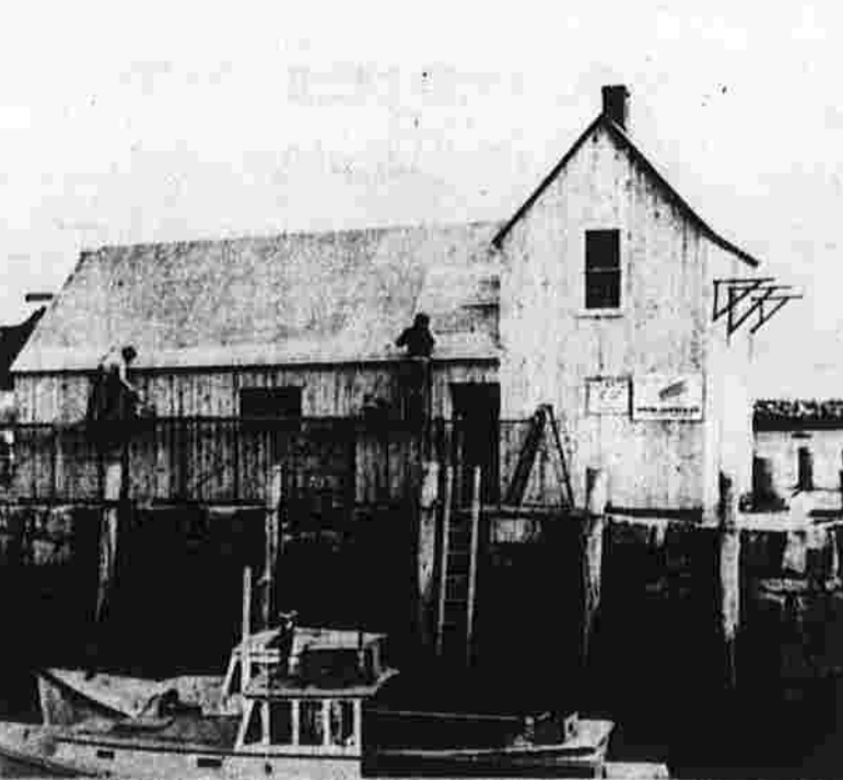
Landmark Nears Completion Shingles are nailed to the roof of Motif No. 1 as reconstruction of the New England landmark nears completion in Rockport, Mass. The original structure was destroyed in the blizzard of Feb. 6, 1978. (UPI photo)
